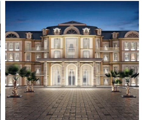
Exterior facades with stucco elements receive a new face.
