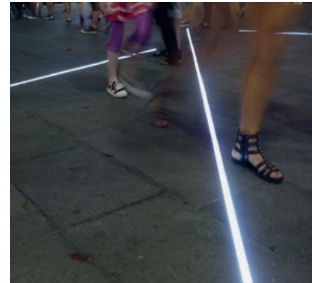
The in-ground steel housing enables a robustness in public areas to walk over.
