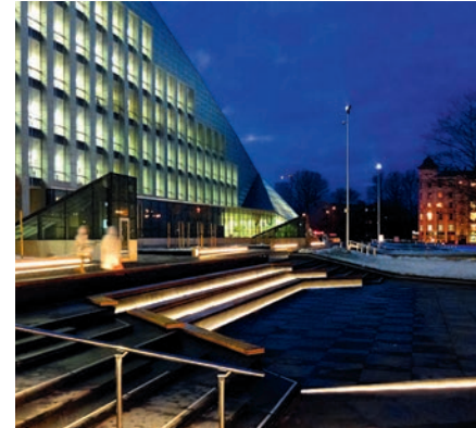
Accenting staircases in public areas create a safe atmosphere and provides orientation.
